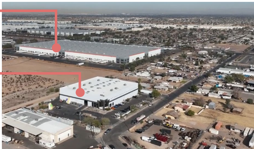
Rectangle owns the 40,000 square foot SSB asset located in the Phoenix, AZ market.
